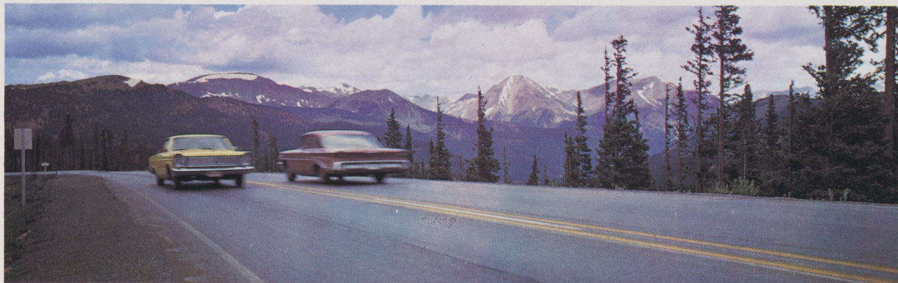
Safe, all-year highways over even the highest mountain passes
