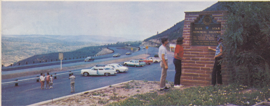
Colorado's Roadside Rest Areas include sheltered tables, grills, restrooms, historical markers, generous parking space
