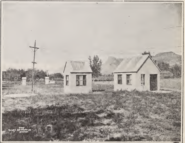
PUMP HOUSE EXTERIOR
