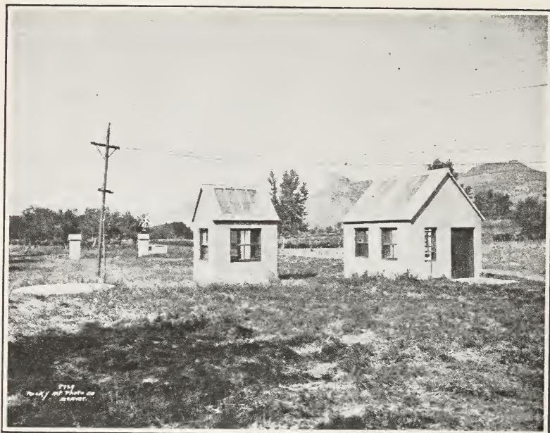
Entrance to Pump House and Well
