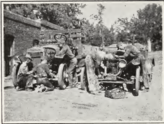
Repairing Truck and Ford
