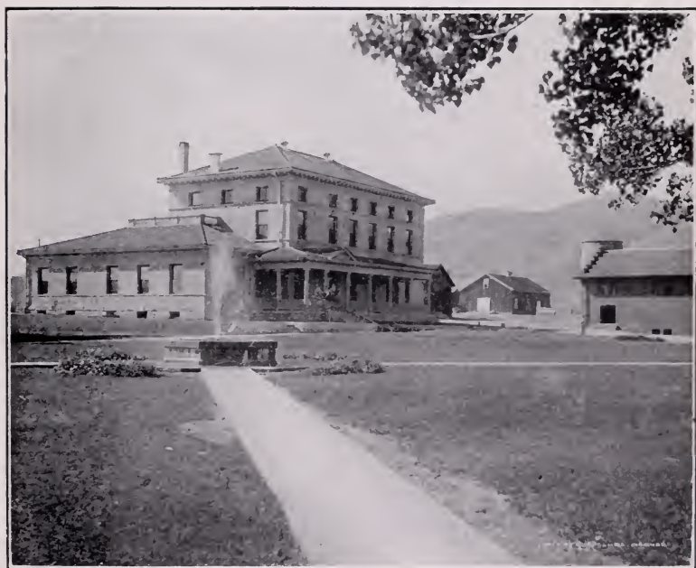
CHAPEL-DINING ROOM BUILDING—SHOWING FOUNTAIN AND WALKS CONSTRUCTED BY BOYS
