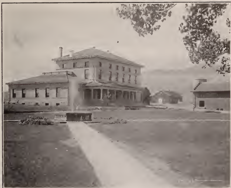
CHAPEL-DINING ROOM BUILDING SHOWING FOUNTAIN AND WALKS RECENTLY CONSTRUCTED
