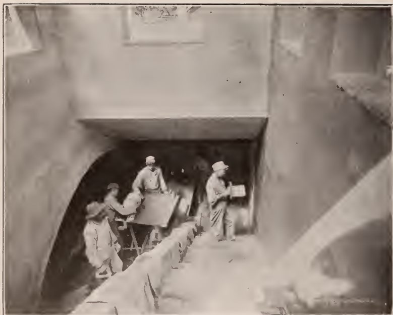
CONSTRUCTING PUMP HOUSE
