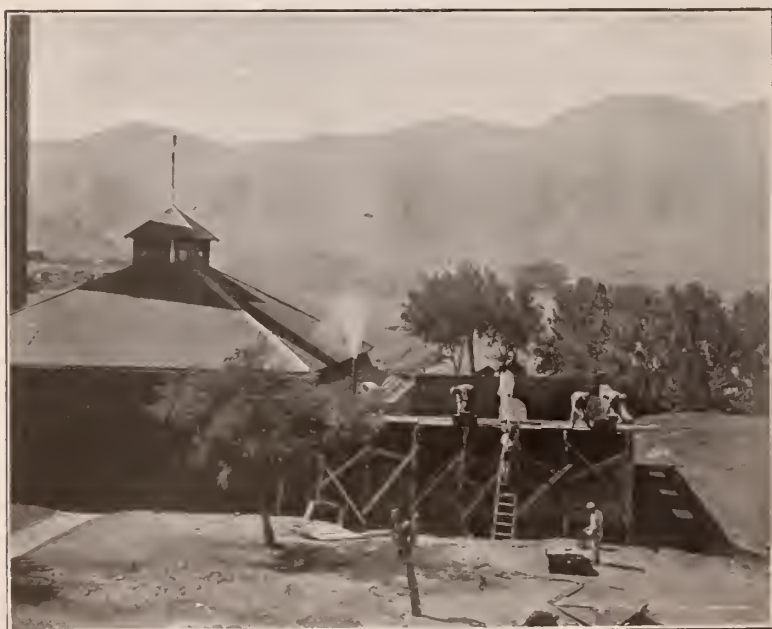
BRICKLAYERS CONSTRUCTING ADDITION TO BOILER HOUSE
