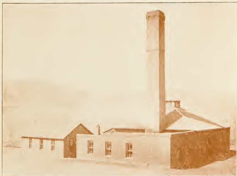
Power House and Machine Shop
