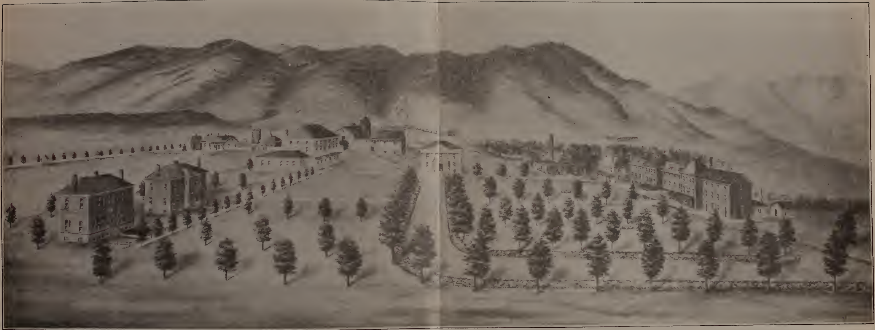
Cottage C Cottage B Steel Standpipe Hospitals Outbuildings Barns Tailor Shop Gymnasium Administration Building Carpenter Shop Power House Officers' Quarters Main Building Ice House GENERAL VIEW OF GROUNDS
