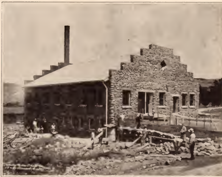
NEW BUILDING FOR LAUNDRY AND TAILORING
