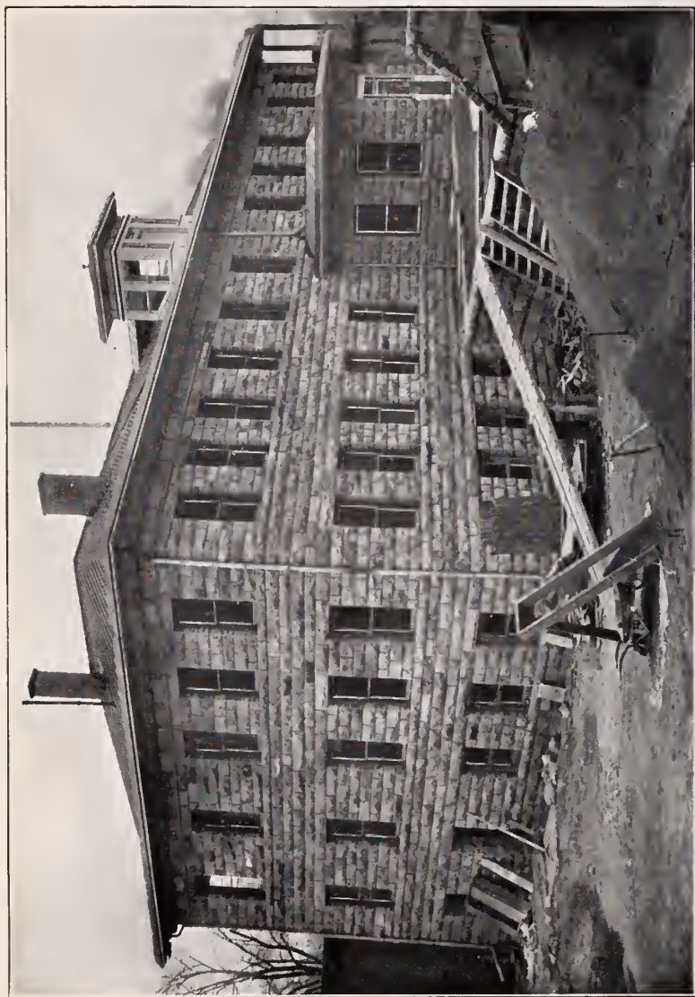
New Administration Building Nearing Completion at Penitentiary; 100 Feet Long, 50 Feet Wide, 3 Stories High. Built of Cut Stone, Steel and Concrete by Prisoners.
