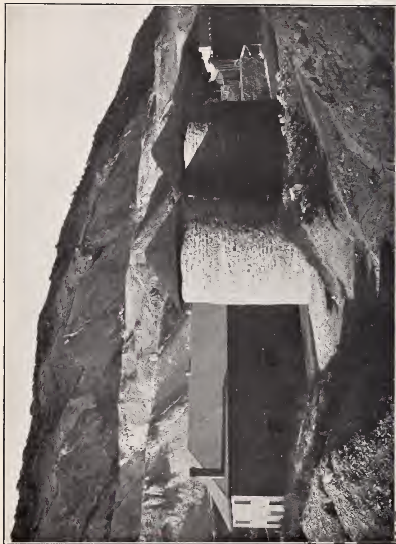
Two Stone Silos, 26 Feet Wide and 31 Feet High, Built by Prisoners at the Penitentiary. They Contain About 300 Tons of Ensilage for Prison Dairy.
