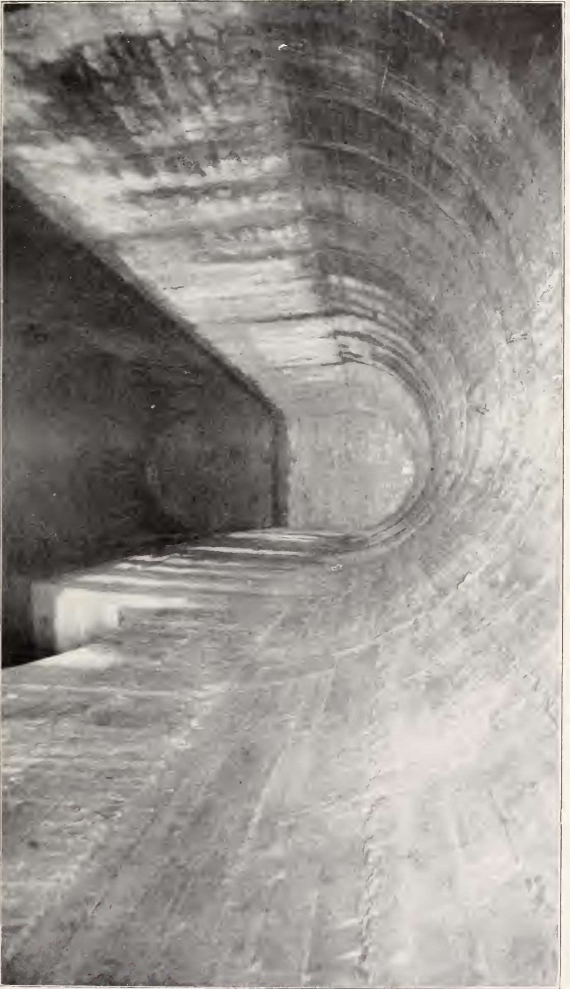
HALE OF UNDERGROUND WELL-RESERVOIR. EACH SIDE 20X100 FEET. INDUSTRIAL, SCHOOL, GOLDEN.
