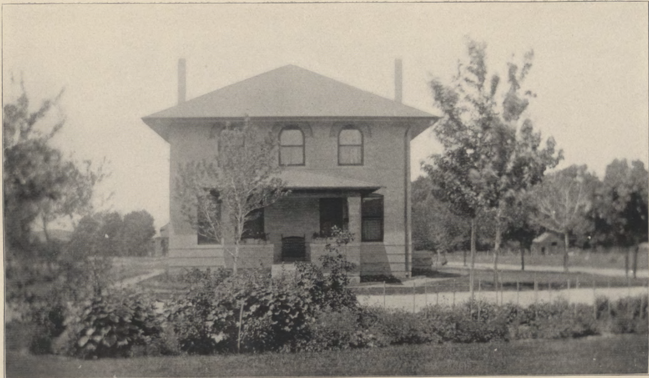
NEW ADMINISTRATION BUILDING, ERECTED 1907. EAST VIEW.
