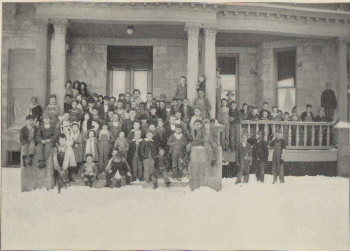
FRONT PORCH, ADMINISTRATION BUILDING.
