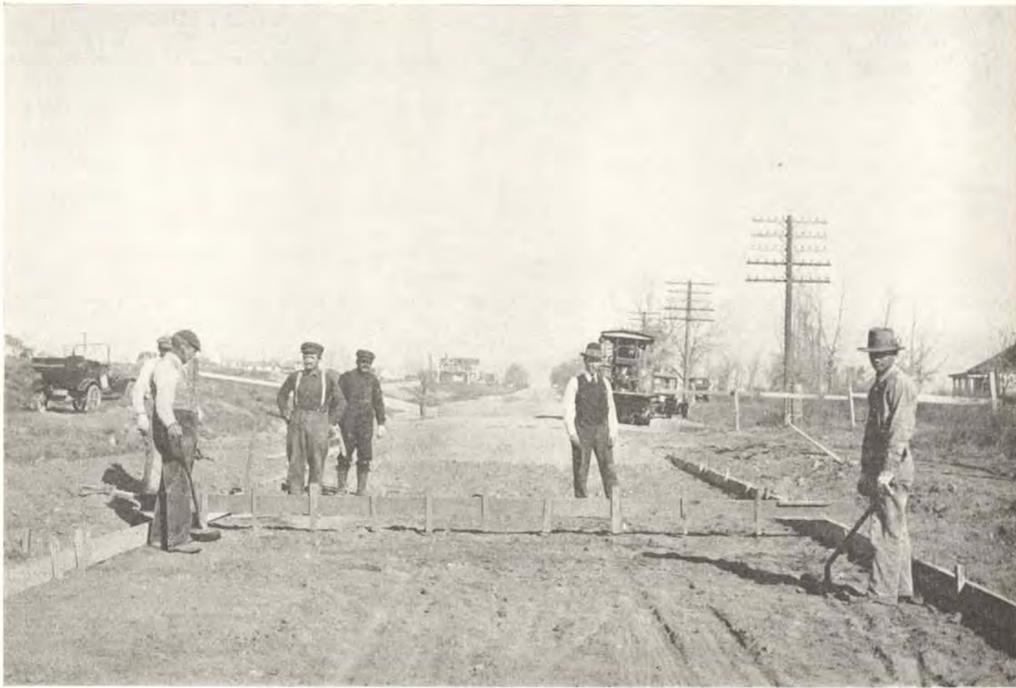
No. 1. Leveling Sub-Grade, Greeley Road.
