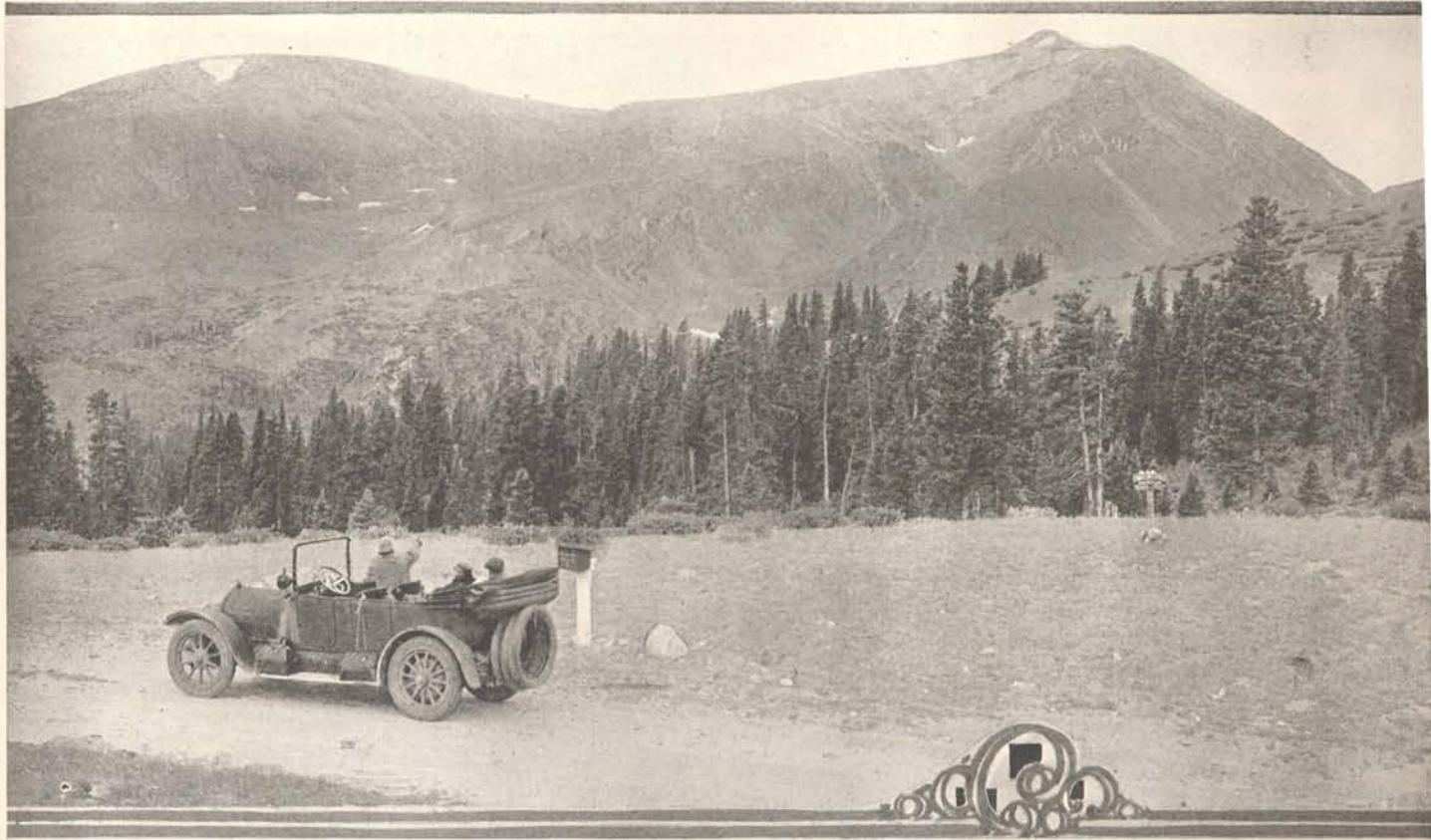
Kenosha Pass. One of the highest and most important passes over the Rockies. Road is being rebuilt here.
