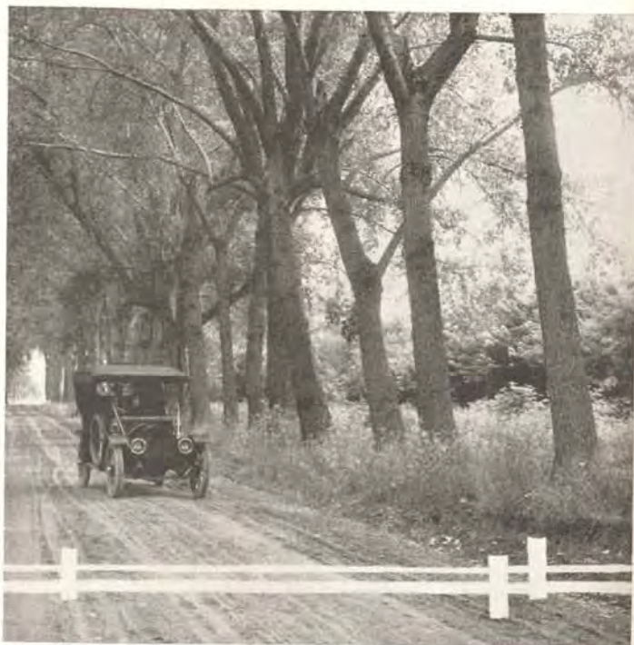
This magnificent line of cottonwoods has been planted along a dirt road, too close to the roadway, two bad points.
