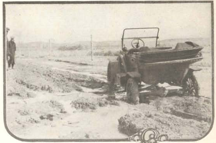
Lack of proper side-ditches is emphasized.
