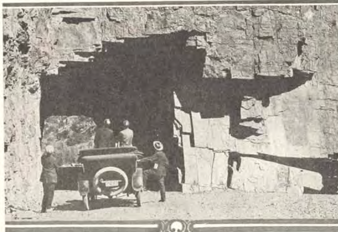
Close-up view of tunnel on the Cache la Poudre Canyon road, Larimer County.
