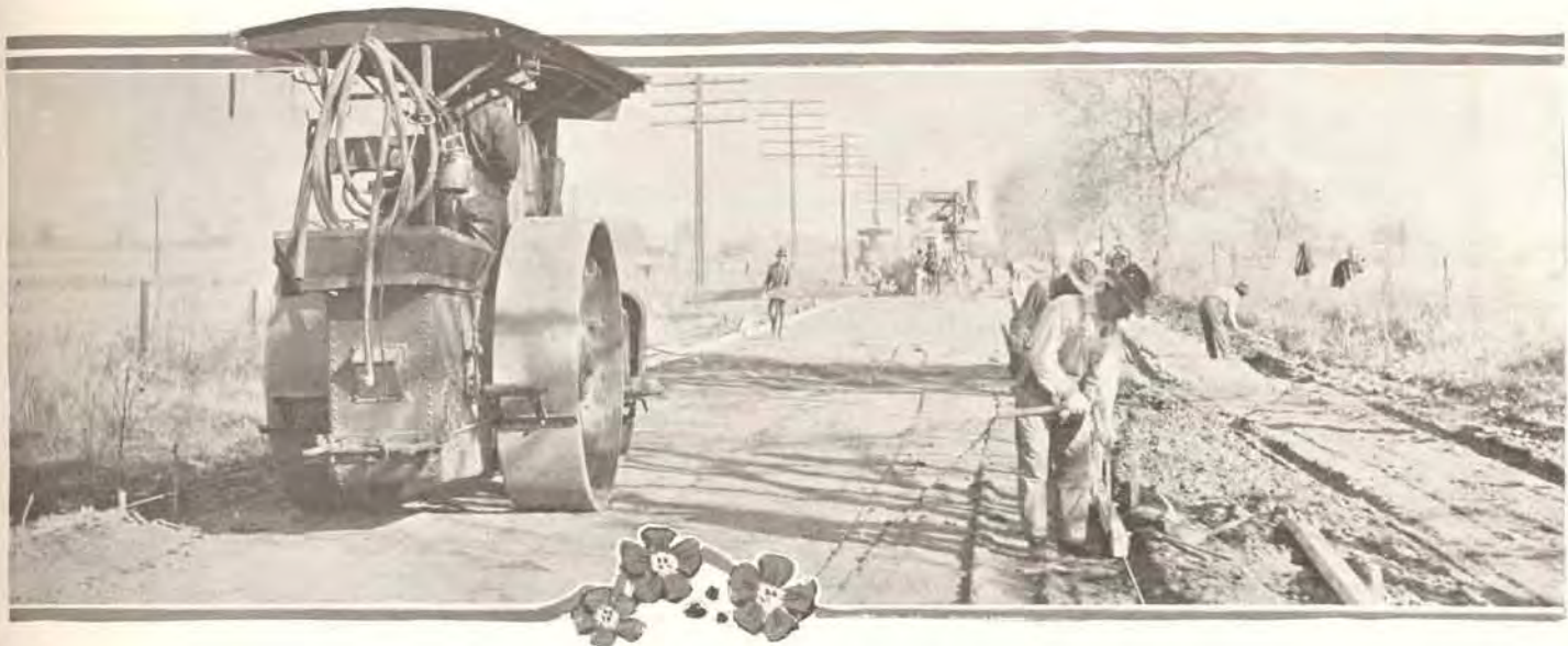
Laying Concrete on the Denver-Golden Road.
