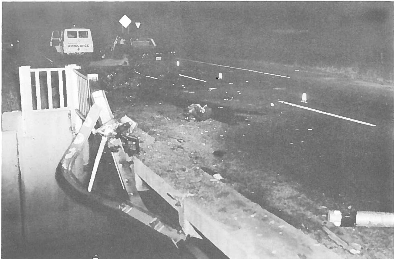
6. High-speed crash into bridge railing at night.
