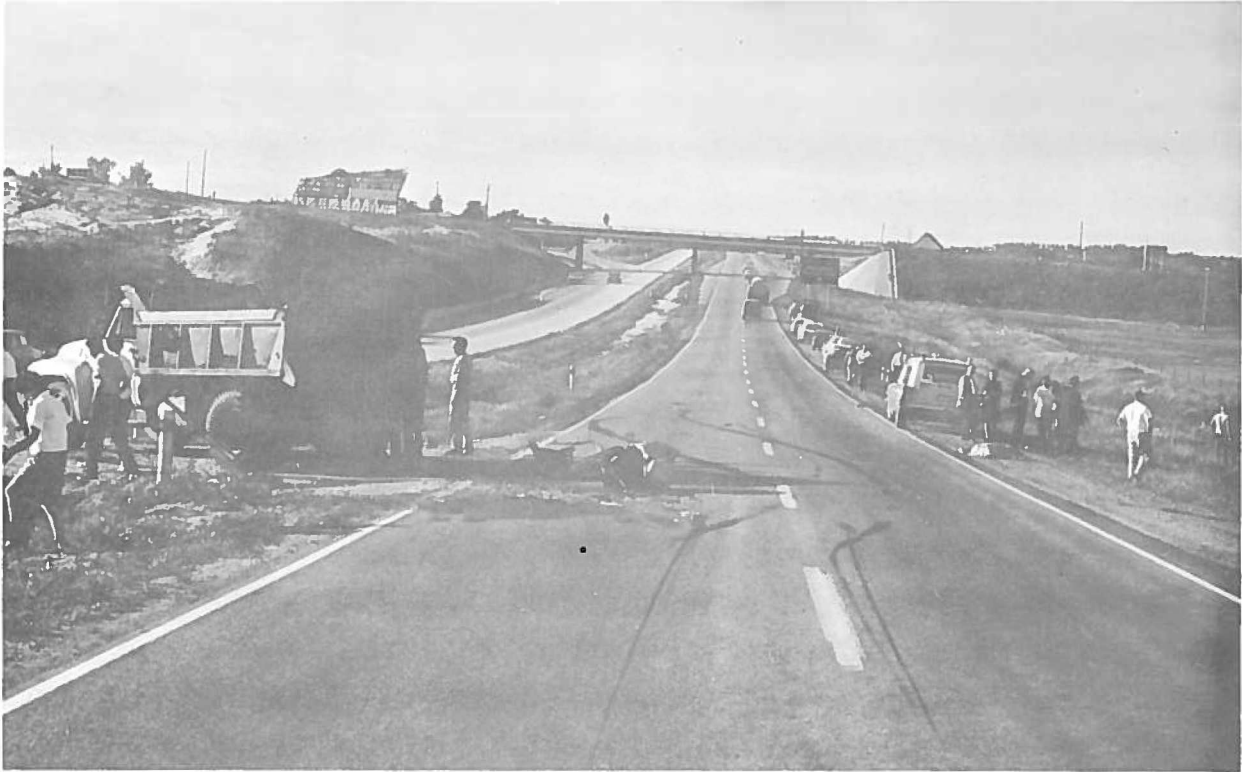
6. U-turn at median crossover causes freeway driver to lose control.
