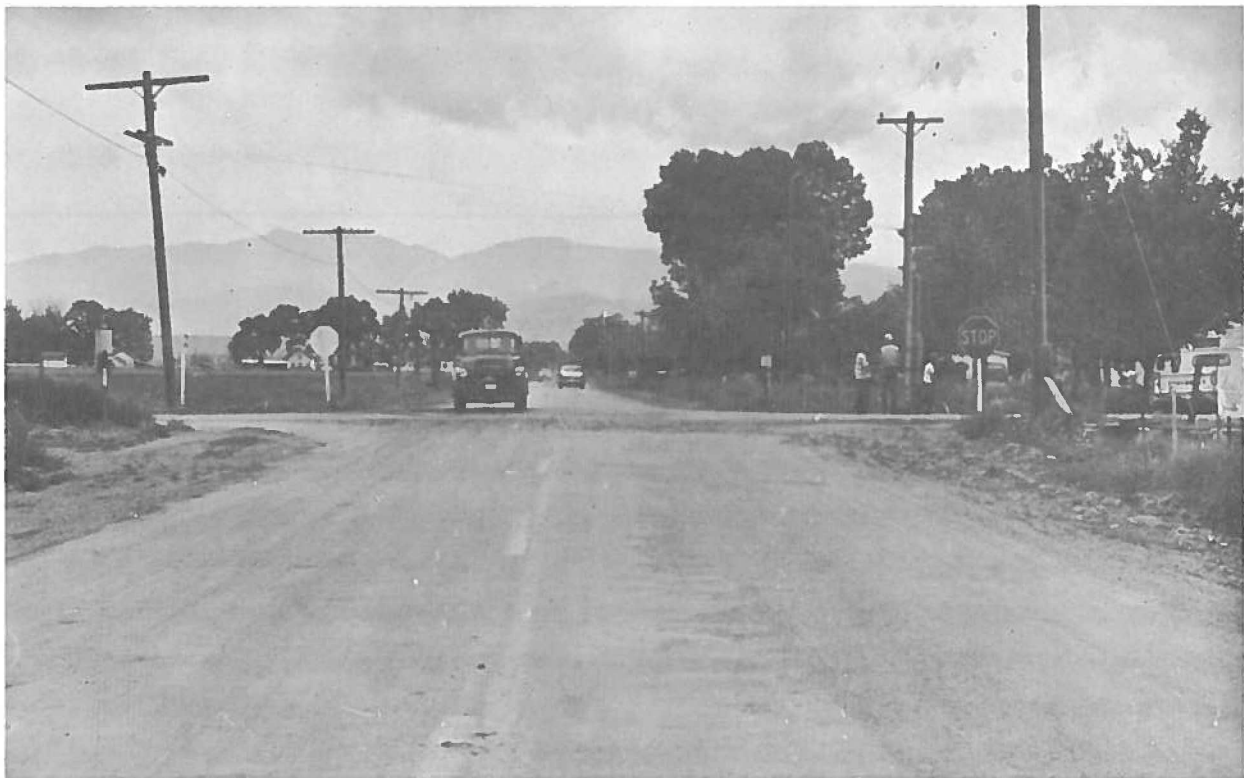
10. Stop sign violation where local road meets State highway.
