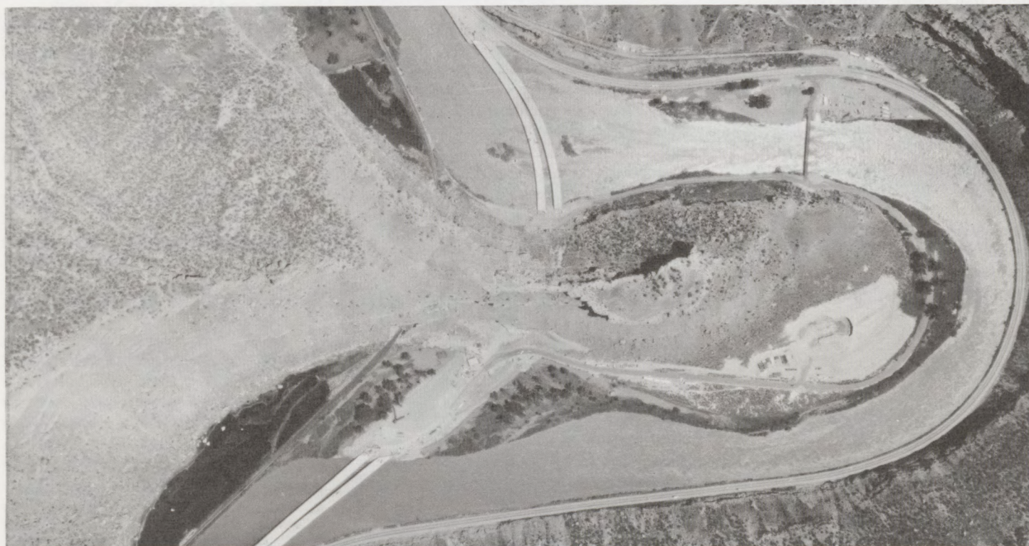
Aerial photo of the "Beavertail" section of I-70 in Debeque Canyon showing work on tunnel and bridges.
