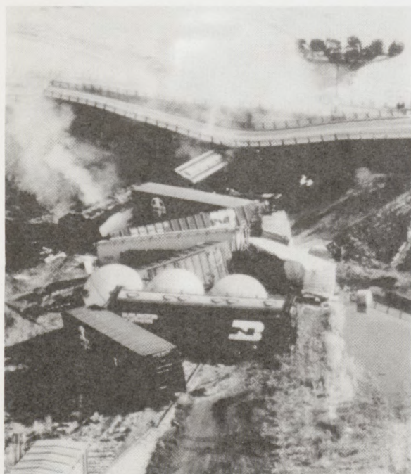
Fortunately, no vehicles were on the twin bridge structures when they were engulfed by the fireball. Temperatures from the fire rose in excess of 1200 degrees, virtually melting the twin U.S. 36 bridges.
