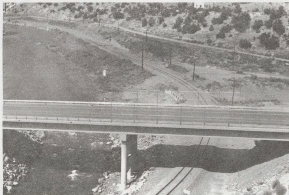
Newly Constructed Bridge
