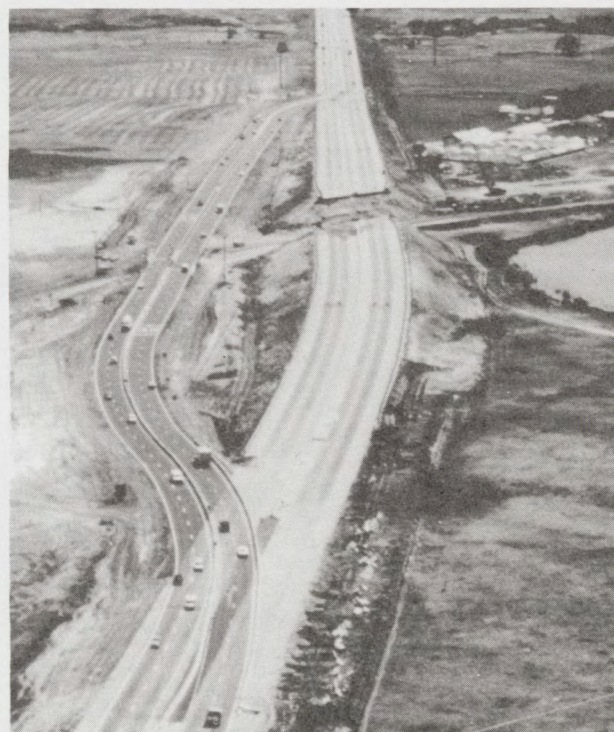
The mile-long temporary four-lane detour crosses railroad tracks just north of the U.S. 36 bridge site. After a new $2 million concrete bridge is opened to traffic December 1, the temporary detour will be removed.
