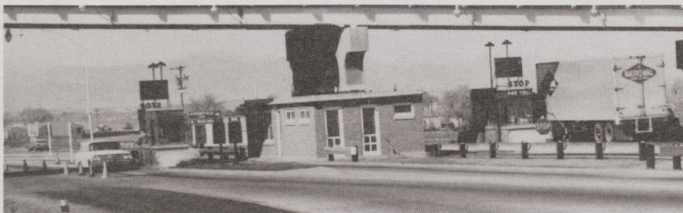
Denver-Boulder Turnpike toll gate, 1957.
