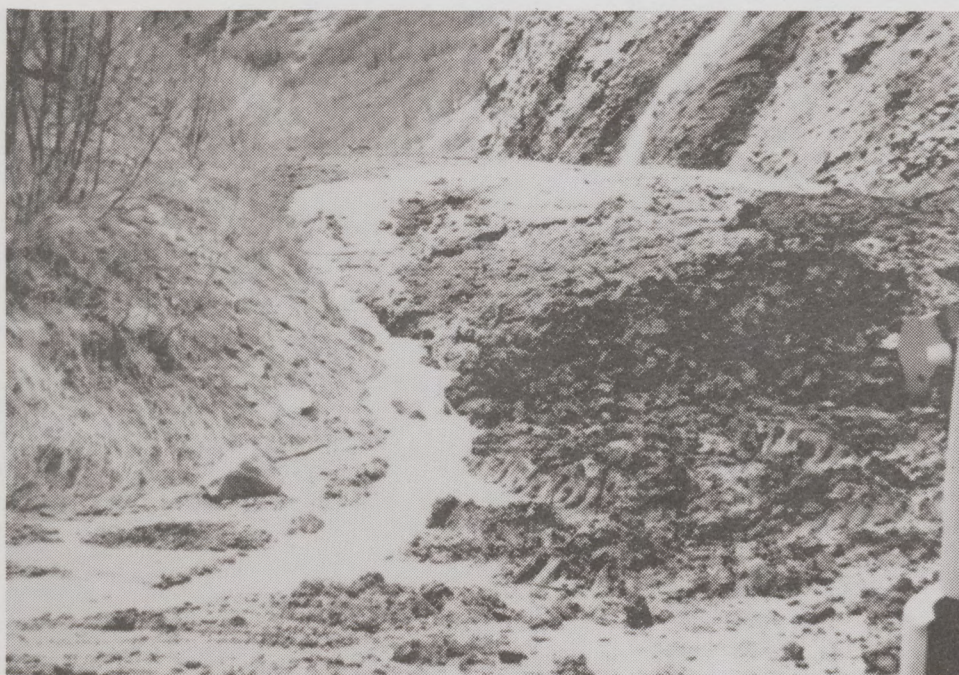
Result of mudslide on S.H. 139, Douglas Pass
