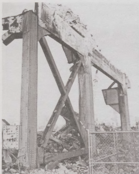
Demolition of Old Colfax Avenue Viaduct
