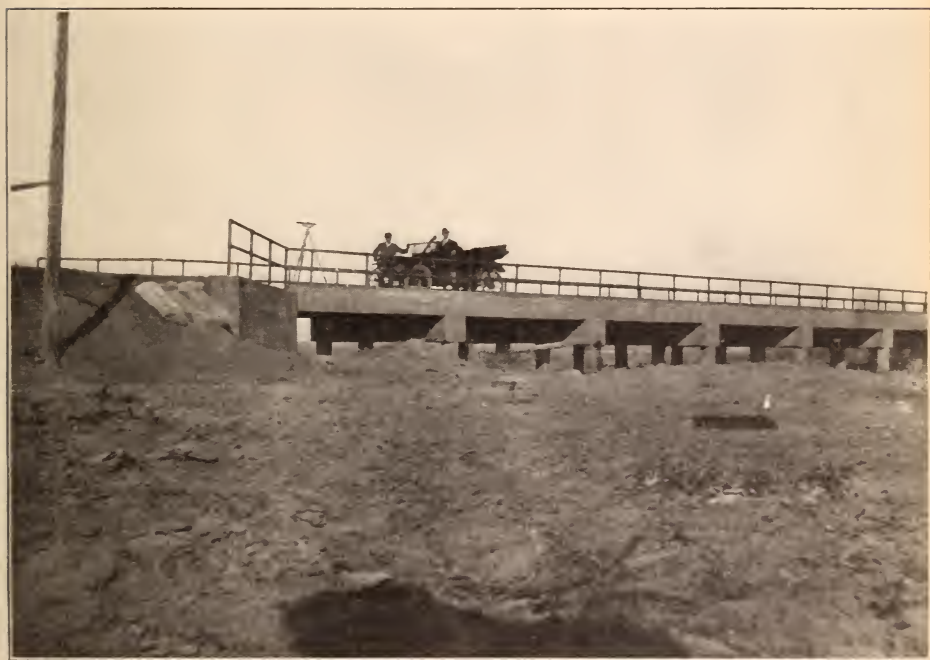
CONCRETE PILE BRIDGE, BIJOU CREEK, MORGAN COUNTY— DENVER-FORT MORGAN ROAD
