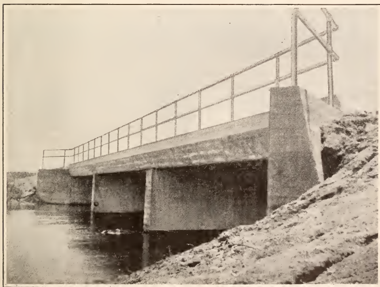
CONCRETE EYE-BEAM BRIDGE OVER SOUTH PLATTE RIVER, NEAR STERLING; FOUR BRIDGES 612 FT. 6 IN. OF OPENING—STATE PRIMARY ROAD NO. 23.
