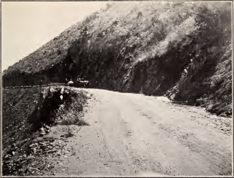
LOOKOUT MOUNTAIN ROAD, JEFFERSON COUNTY, MOUNTAIN PARK COMMISSION OF DENVER, CLEAR CREEK SIDE— STATE PRIMARY ROAD NO. 21.
