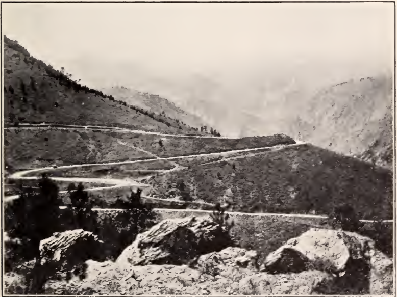
LOOKOUT MOUNTAIN ROAD, SHOWING HAIRPIN CURVES TOWARD TOP (MAXIMUM GRADE 6 PER CENT)—STATE PRIMARY ROAD NO. 21.
