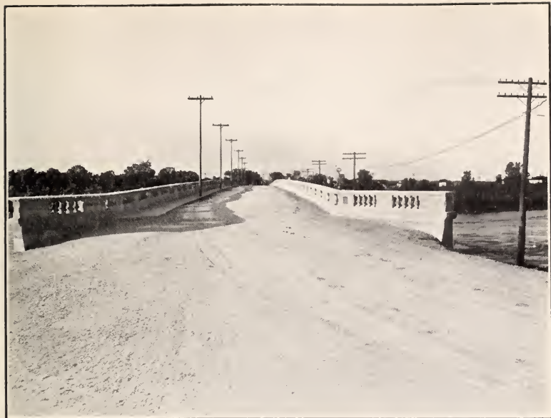
REINFORCED CONCRETE ARCH BRIDGE AT LA JUNTA, OVER ARKANSAS RIVER—STATE PRIMARY ROAD NO. 6.
