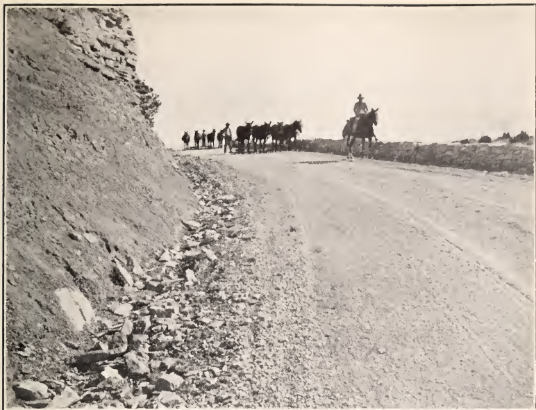
DRAGGING PUEBLO-BEULAH ROAD, CONVICT LABOR—STATE SECONDARY ROAD NO. 7 s.
