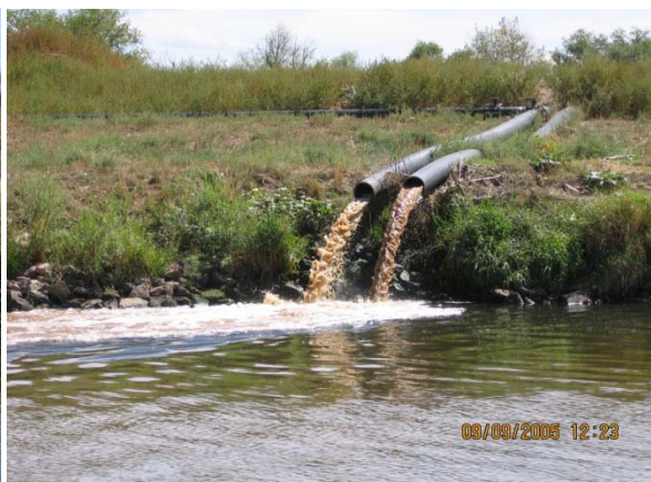
Discharge out of compliance
