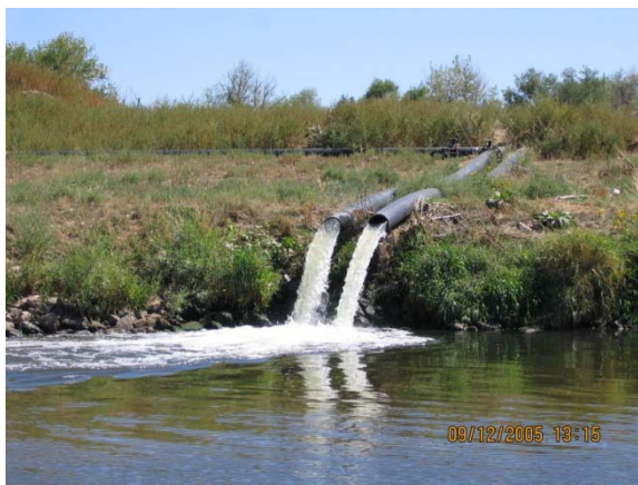
Discharge in compliance
