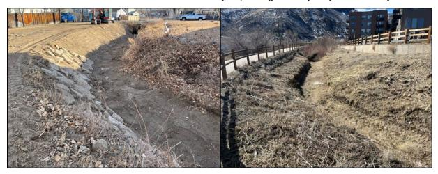
Left: Vegetation removal, ditch shaping, and rip rap placement to reduce erosion near W. 75<sup>th</sup> Way, right: Vegetation removal Basecamp in Golden
