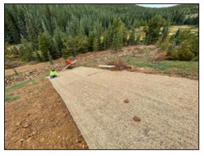
Snowden Mine: Contractors laying erosion control matting across reseeded slopes.
