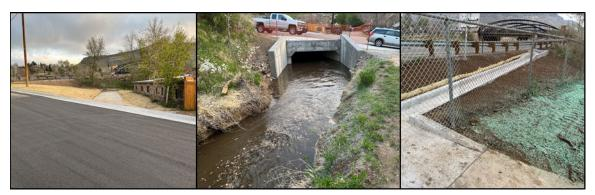
Left: Arapahoe culvert replacement and extension, middle: Arapahoe culvert inlet, right: Highway 52 exit ramp storm water diversion channel
