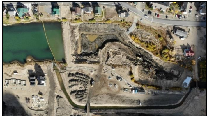
Georgetown Lagoon dredging project
