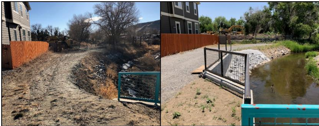
Figure 5. Church Ditch Easement Before (left) and After (right) Improvements
