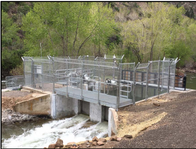
New Church ditch headworks structure.
