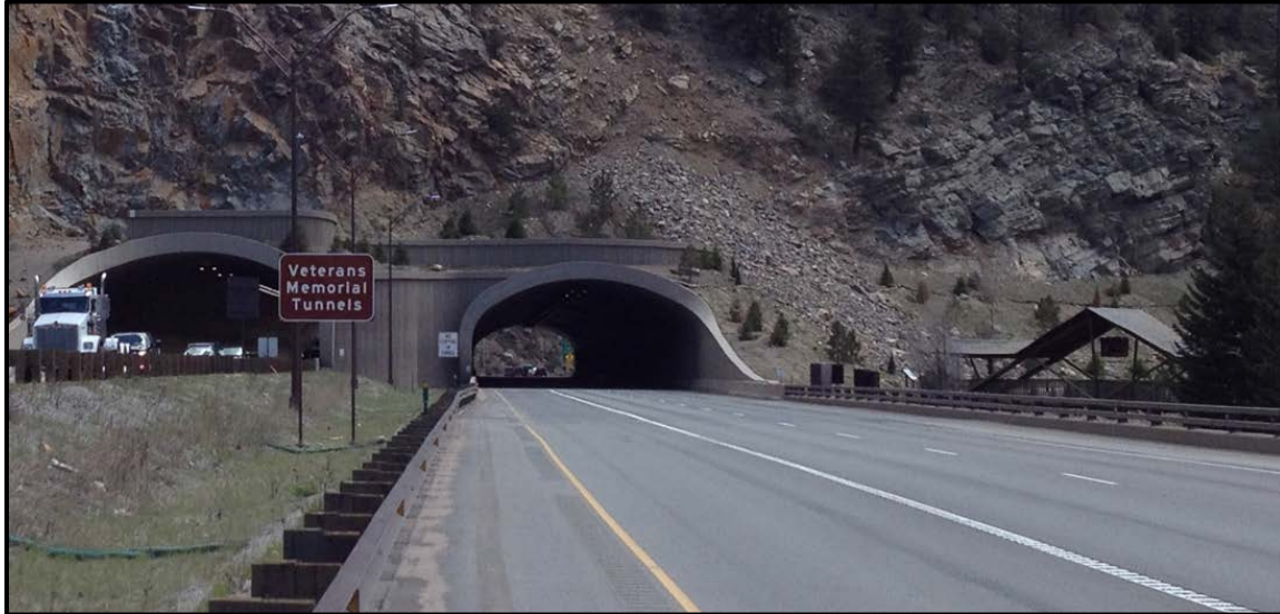
Eastbound Twin Tunnels After Completion (Photo Credit: CDOT)
