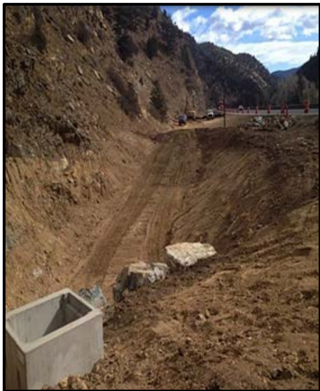
Construction of Detention Basin for Clear Creek Sediment Control Project
