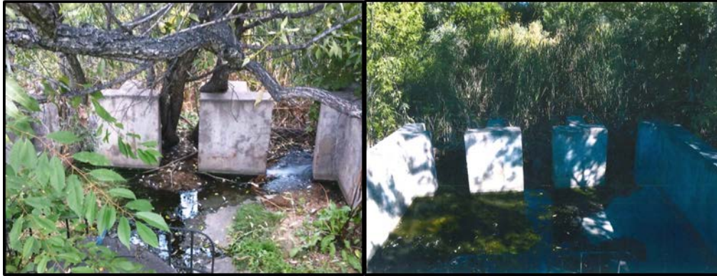
Stormwater Structure Before (Left) and After (Right) Maintenance Activities
