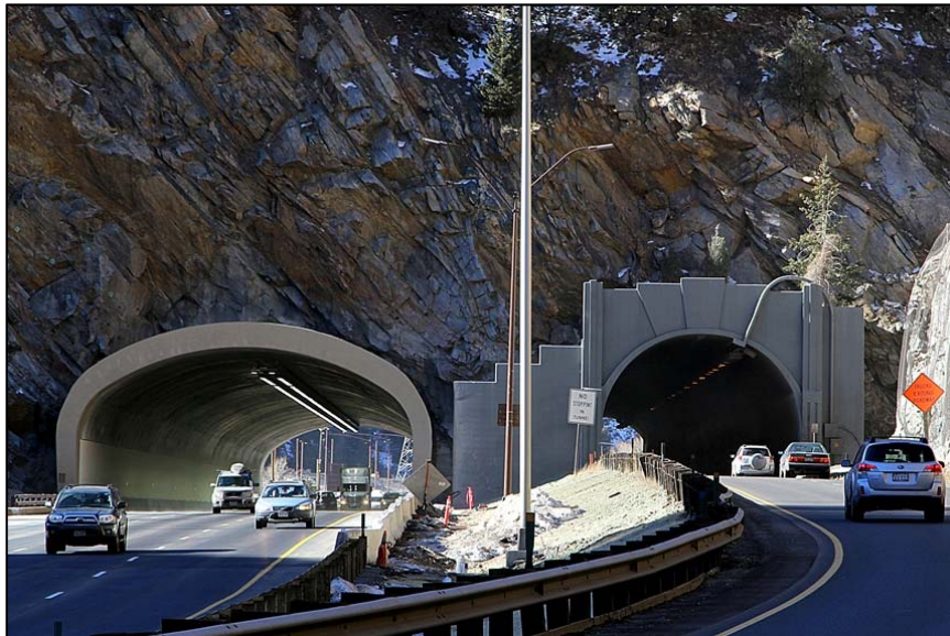
Figure 19. Twin Tunnels: Completed Wider Eastbound Tunnel (left), To-be Widened Westbound Tunnel (right); Image from: http://www.coloradodot.info/projects/i70towntunnels
