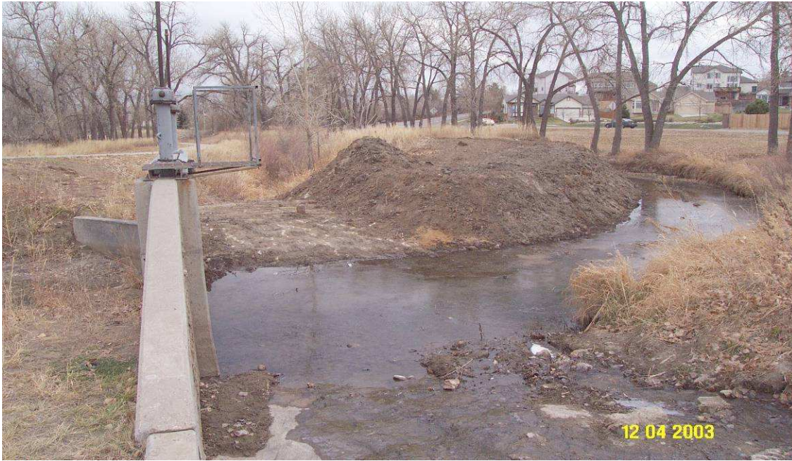
Figure 26. Old ditch structure. Ditch in center of the photo with Little Dry Creek inflows on bottom right.
