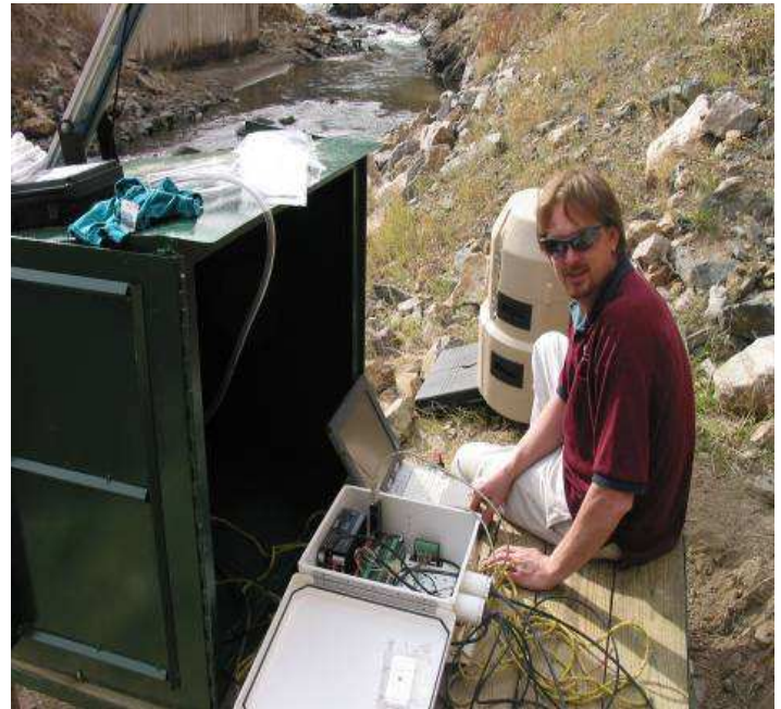
Figure 1. Monitoring Station Installation
