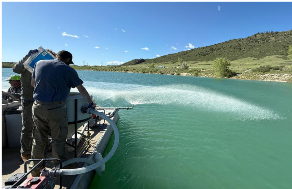
Image 1. Phosphorus sequestration application at Big Soda Lake, 2025.
