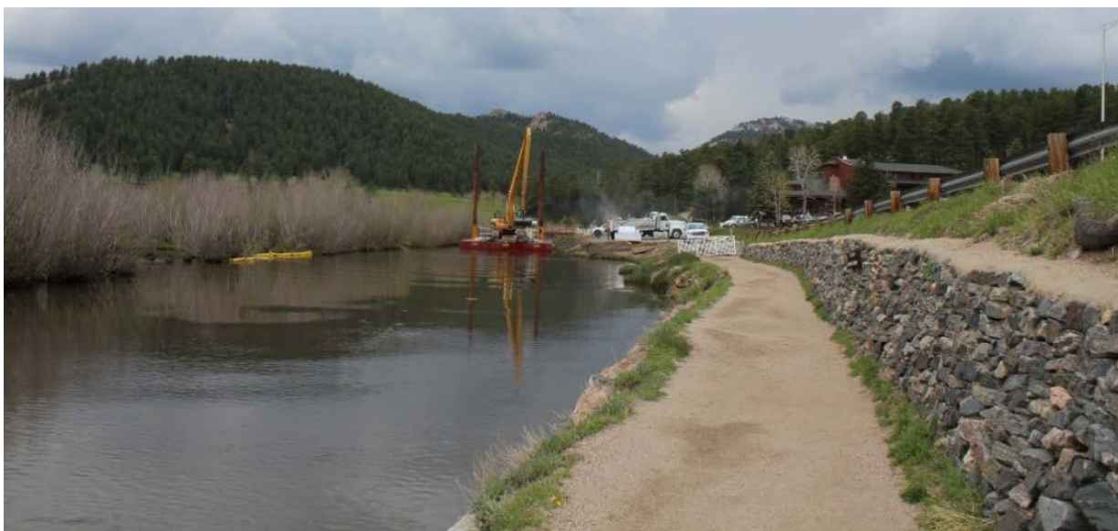
Figure 33 Dredging in Channel
