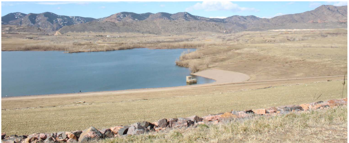
Figure 32 Corps of Engineers Dam Improvements
