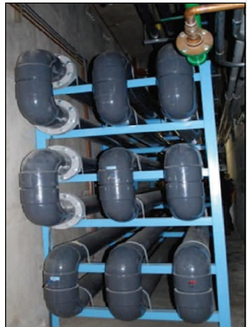
Example of a pipe loop contactor
