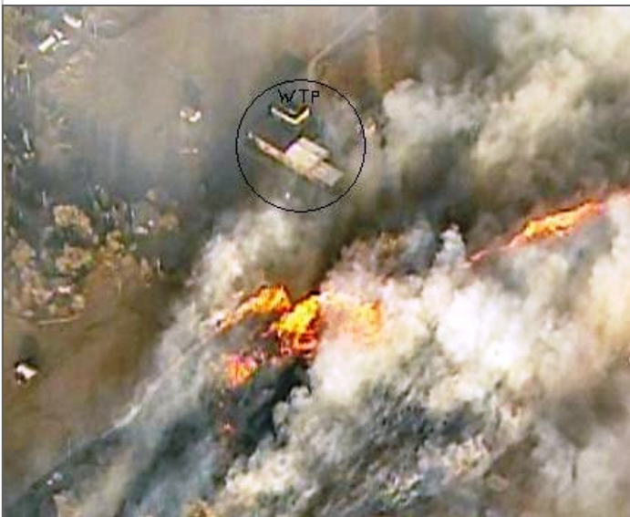
Boulder county water treatment plant surrounded by fire during 2009 fire season.
