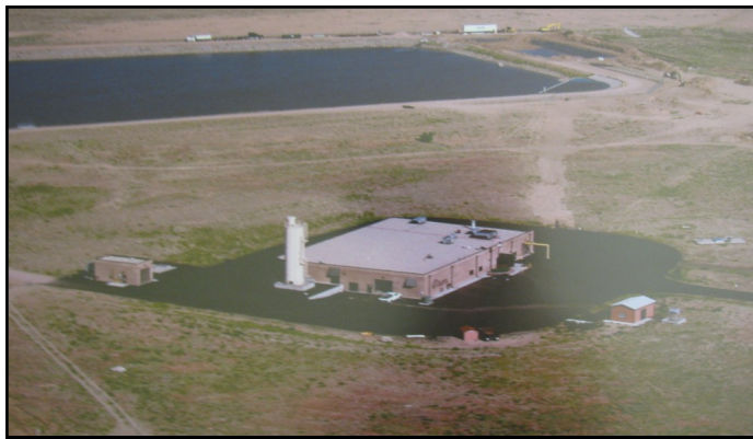
A bird's eye view of Fort Morgan's water treatment
