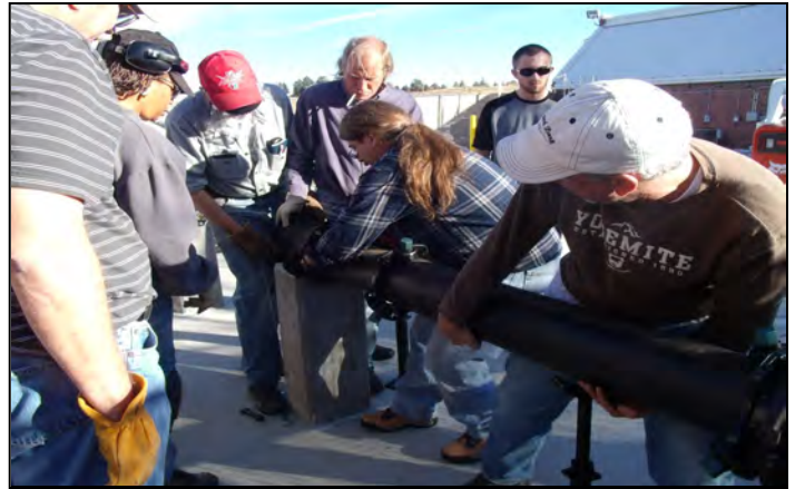
Red Rocks Community College students constructing hands-on components of the training center
