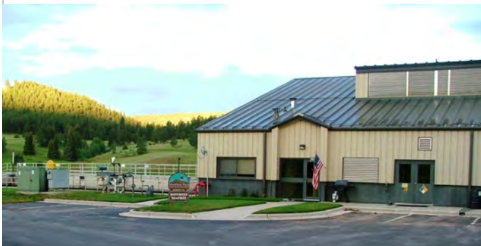
Woodland Park wastewater treatment plant
