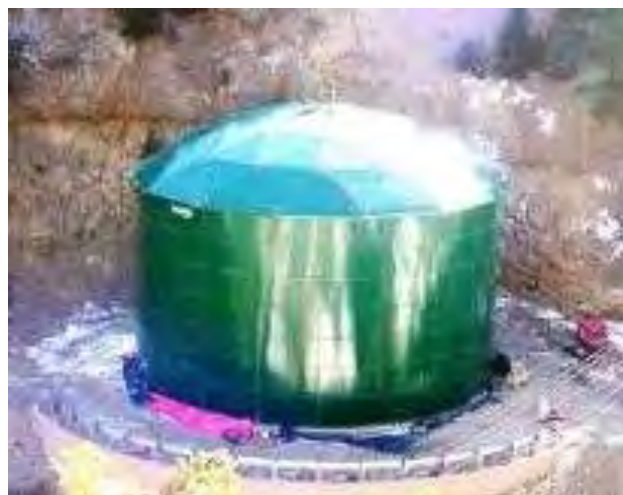
Georgetown water storage tank
