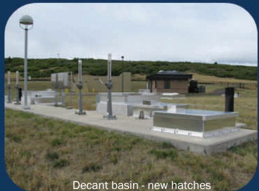
Decant basin - new hatches
