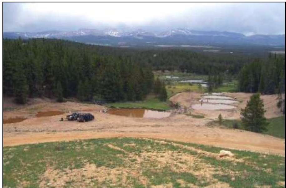
View of mitigated mine waste footprints and retention ponds at Dinero
