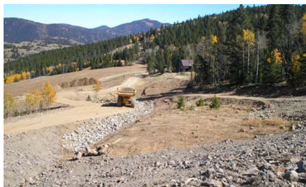
Construction of a new repository cell will start this fall.
