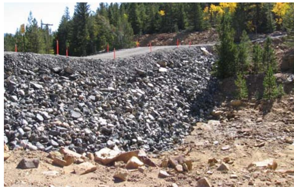
The Nevada Gulch Sediment Retention Basin was constructed in 2007 as part of OU4, Phase I.
