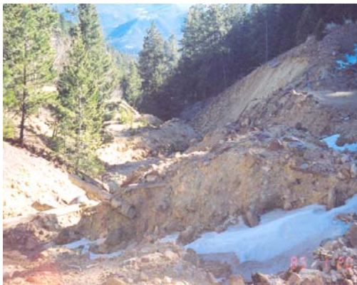
The Diamond Joe Waste Rock Pile (left), Trio Waste Rock Pile (right) and other mine waste rock piles had eroded into the Virginia Canyon channel, which created the need for this summer's removal action by the U.S. Environmental Protection Agency.
