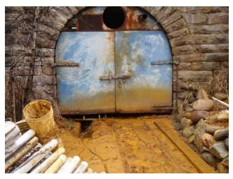
The Big Five Tunnel is located on the west end of Idaho Springs. Normally, mine drainage flows into the trench to the left of the door at 20-30 gallons per minute.
