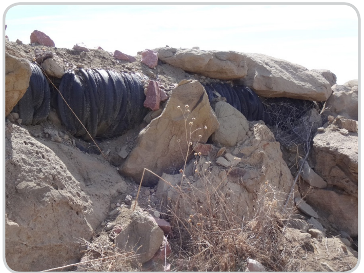
The picture on the left shows the tire bale fence burning during the El Paso County tire bale fire. On the right we see tire bales encased in dirt and rock that did not burn.
