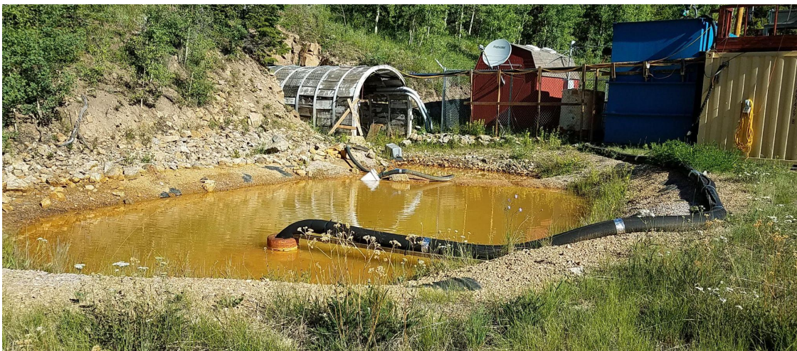
An upper settling pond outside Big Five Adit Portal at the Captain Jack Mill Superfund Site
