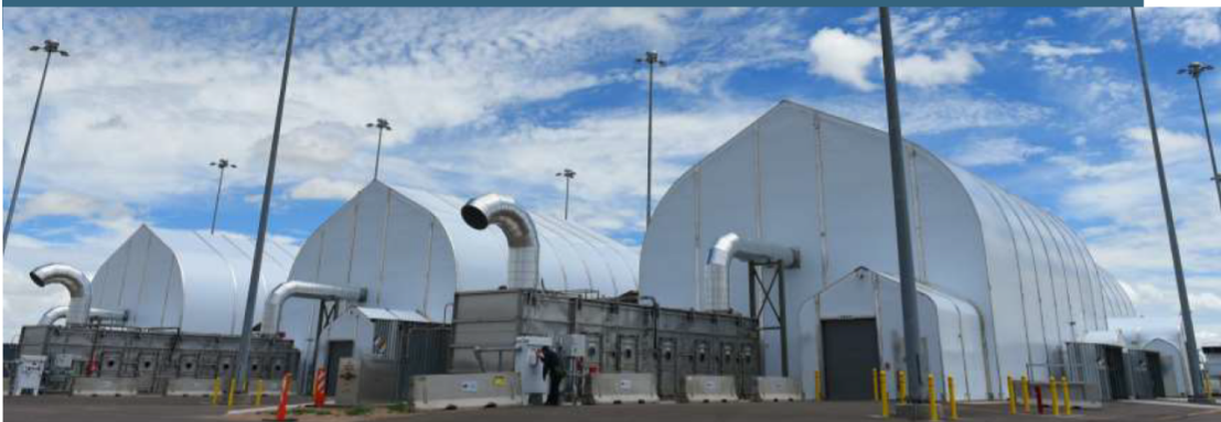
Completed construction of Static Detonation Chamber (SDC) units
