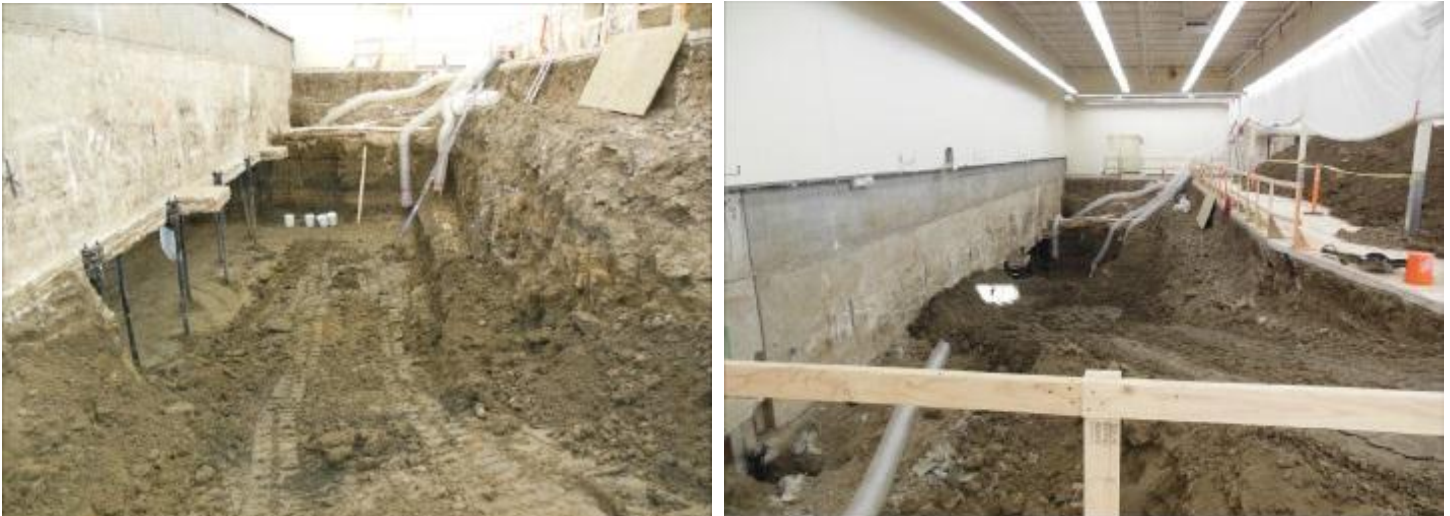
Interior excavation of soils at former Dependable Cleaners
