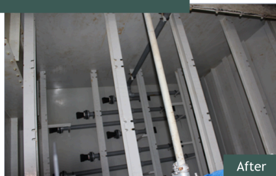
Immobilized Cell Bioreactor media cleanout
