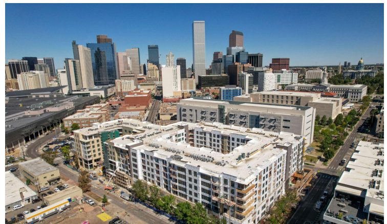
Redevelopment project at a former orthodontics manufacturing facility resulting in the excavation of contaminated soil and additional groundwater remediation.
