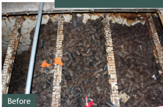
Immobilized Cell Bioreactor media cleanout
