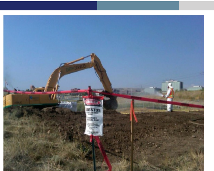
A photo of the remediation of asbestos contaminated soil at the Denver Federal Center
